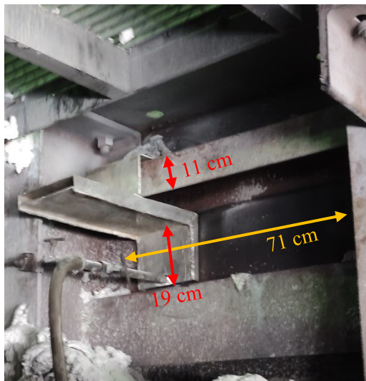
Figure 3. SHE installation at pot sidewall.
